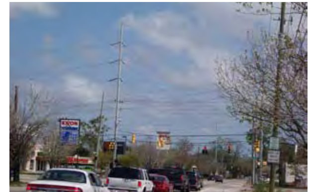
Overhead utility lines will be relocated
