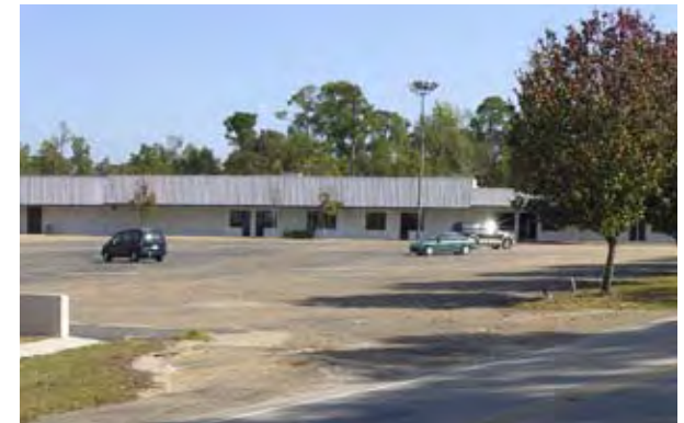
Strip commercial development along Museum Drive
