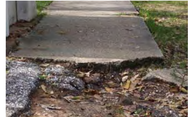
Sidewalks will be reconnected to improve walkability
