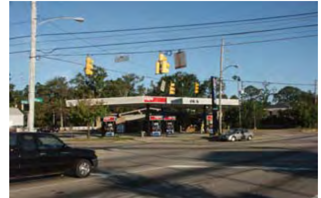
Gas station on the NW corner of Old Shell and McGregor
