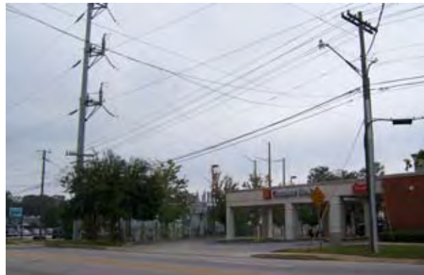
Power lines and utility poles dominate the roadway
