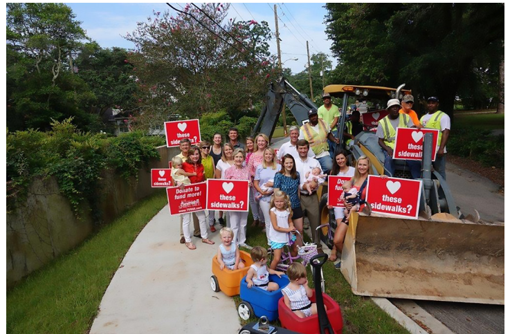
It takes a Village to build sidewalks!
