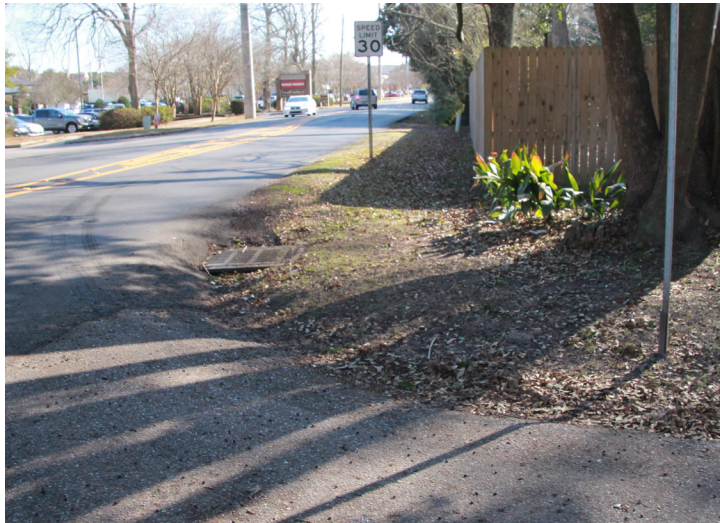
Need for curb, gutter, updated drainage and sidewalks on North McGregor Ave.
