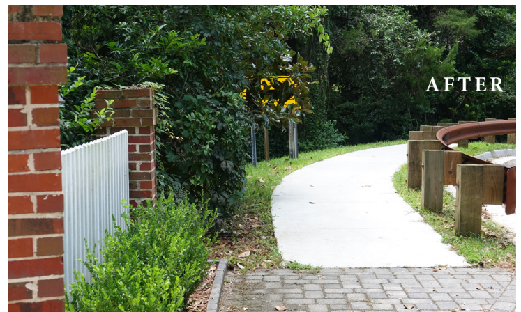
Before and After of East side South McGregor Ave. completely transformed last year
